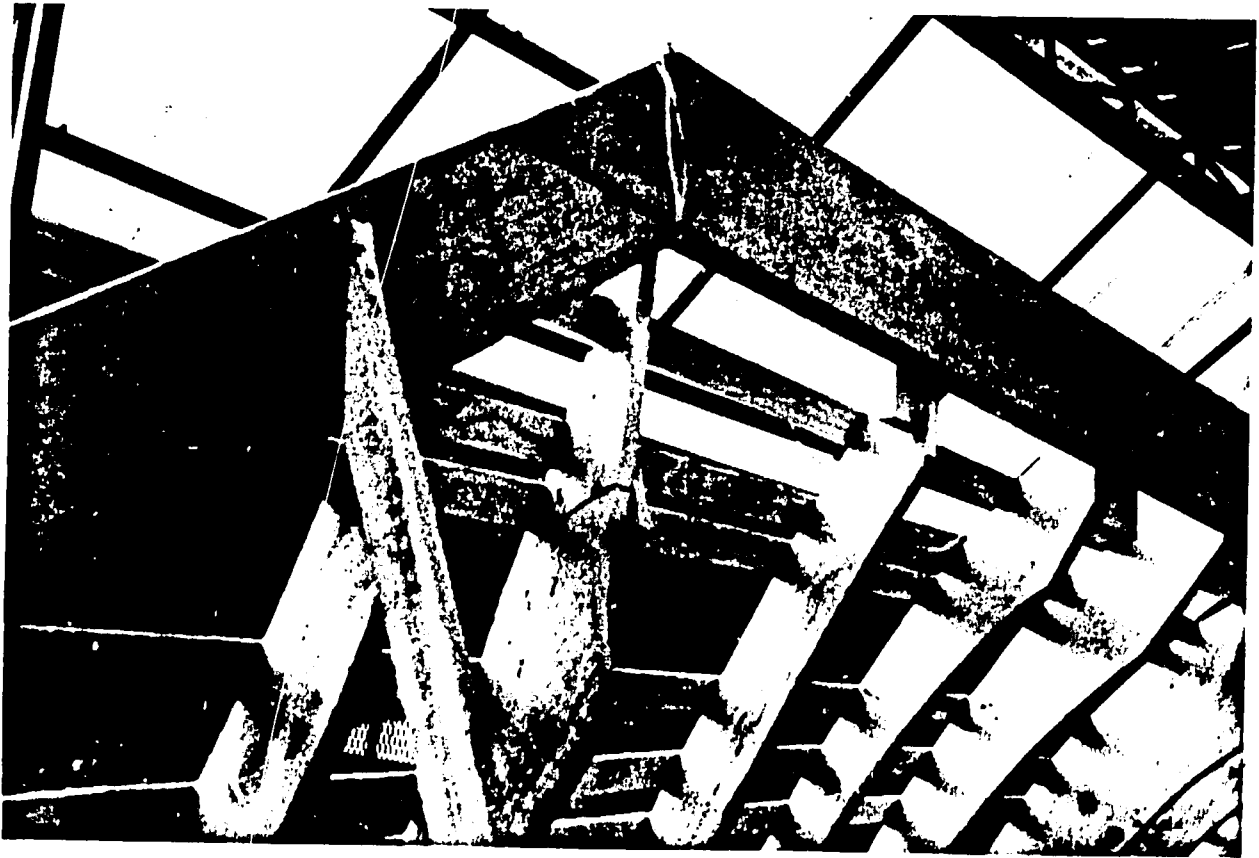
PHOTO 29 DETAILED VIEW OF BOW SECTION WITH ONE SIDE OF FRAMES AND FAIRING STRIPS IN PLACE
