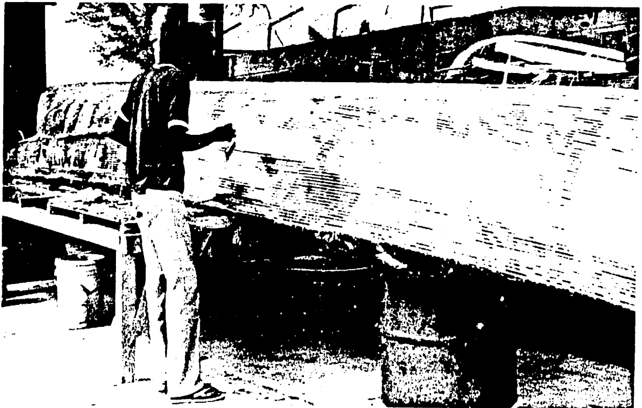
PHOTO 20 RESIN BEING APPLIED TO C-FLEX
