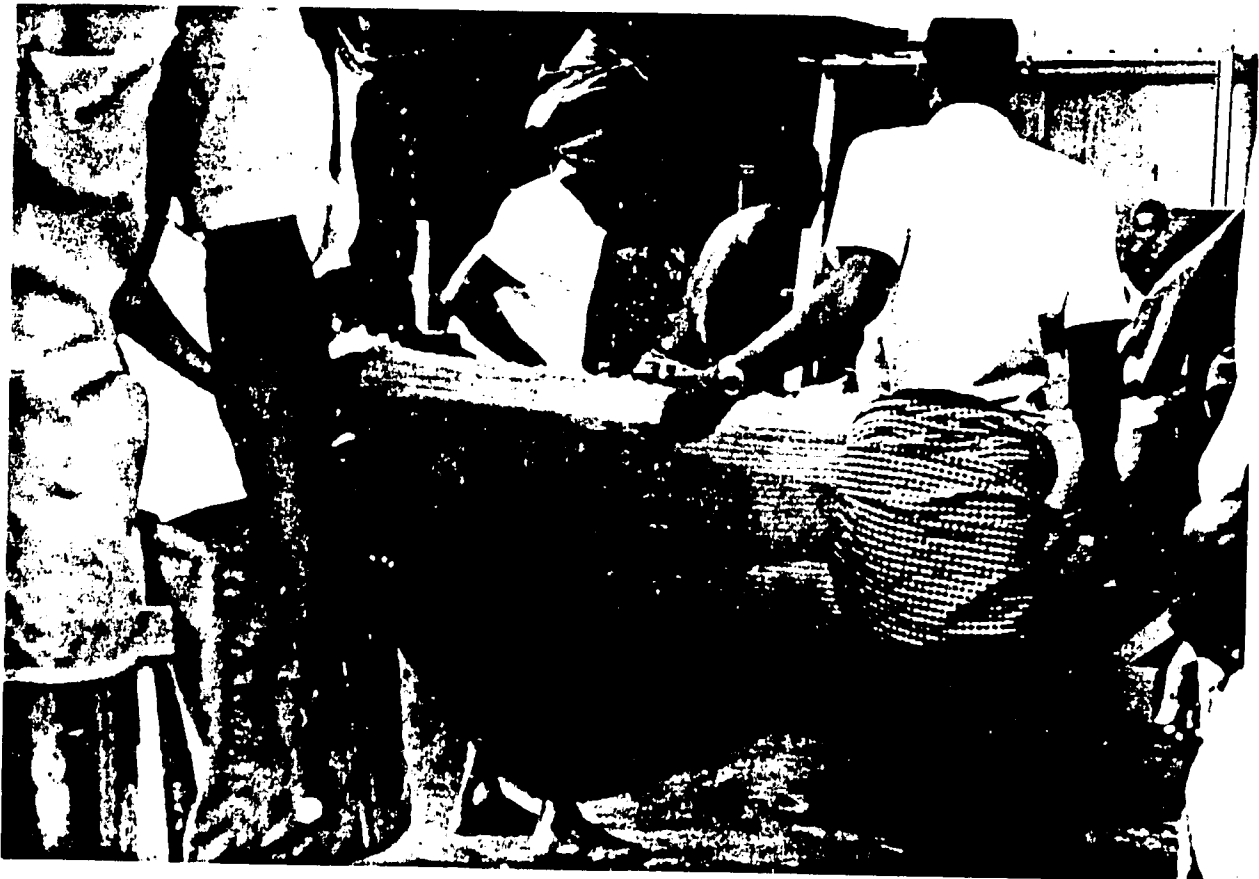
PHOTO 22 PLACING NEW HULL IN CRADLE FOR COMPLETION OF INTERIOR
