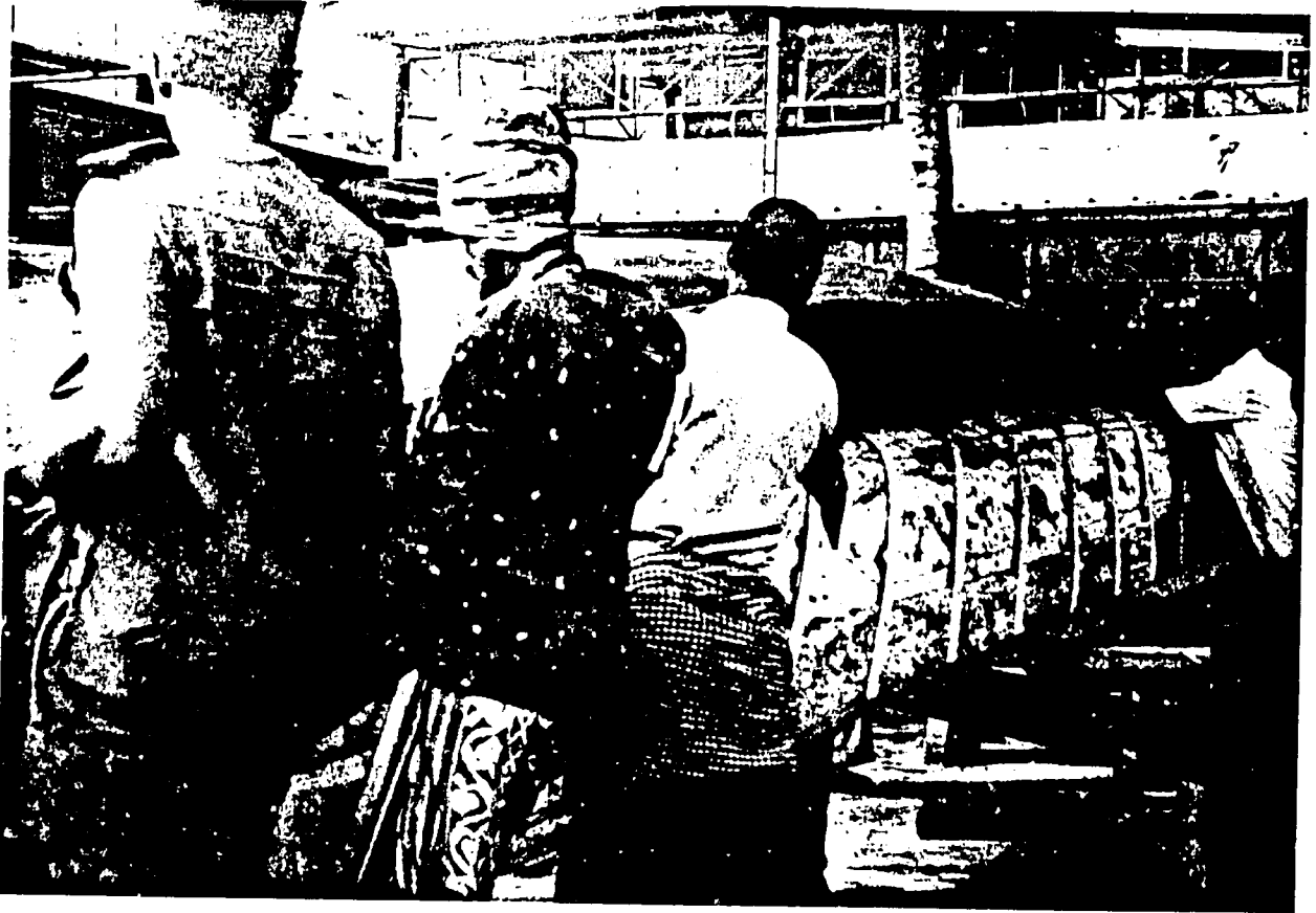
PHOTO 21 LIFTING OFF THE NEW HULL
