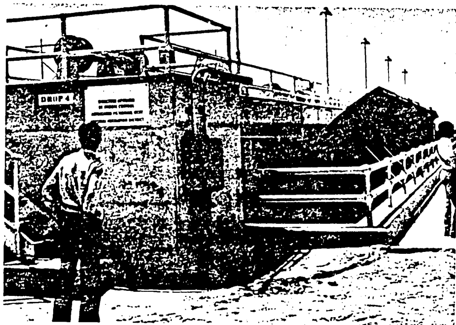
Left, the Solano MOD-2 wind machine is rated at 2.5 MW. The rotor — 91 meters tip to tip — is supported on a 59 meter steel tower. Above, the Drop 4 low-head hydropower plant on the All American canal in southern California. Two vertical axis turbines generate 20 MW from the 15 meter drop.
