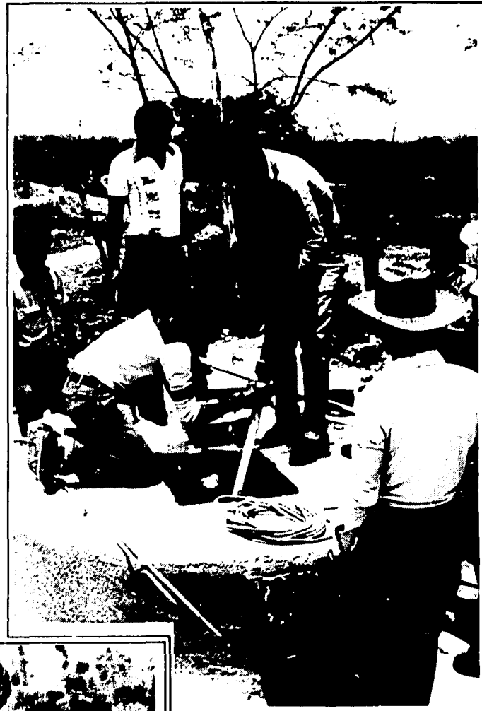
Attaching Roboscreen filter to deep well cylinders.
