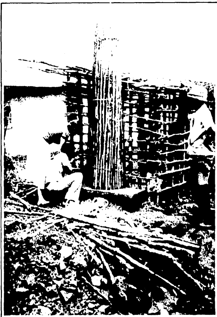
Vent pipe during construction.
