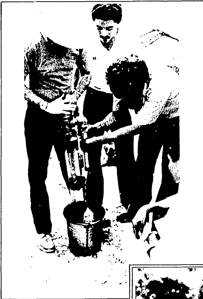
Use of the transparent demonstration pump cylinder proved to be a valuable aid in training caretakers and promoters in troubleshooting and repair techniques.
