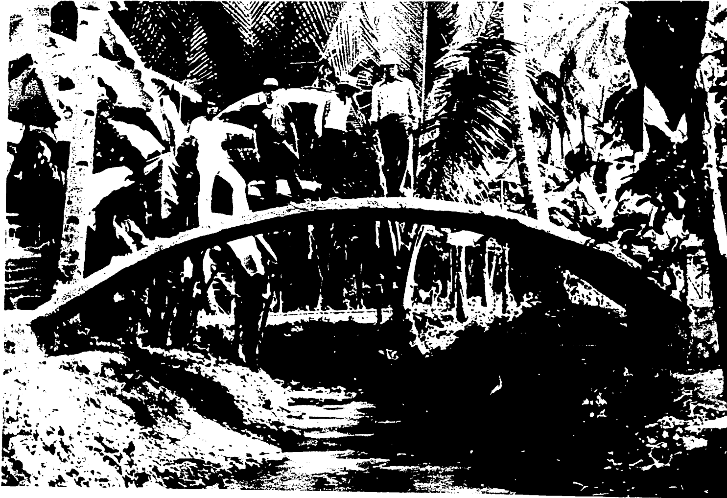
Figure 21 (FERROMBU) BRIDGE; BAMBOO REINFORCED COMBINED WITH CHICKEN WIRE SPAN 9 M; 1,5 M WIDTH; CURVED SHAPE PREVENTS LOSS FROM FLOOD
