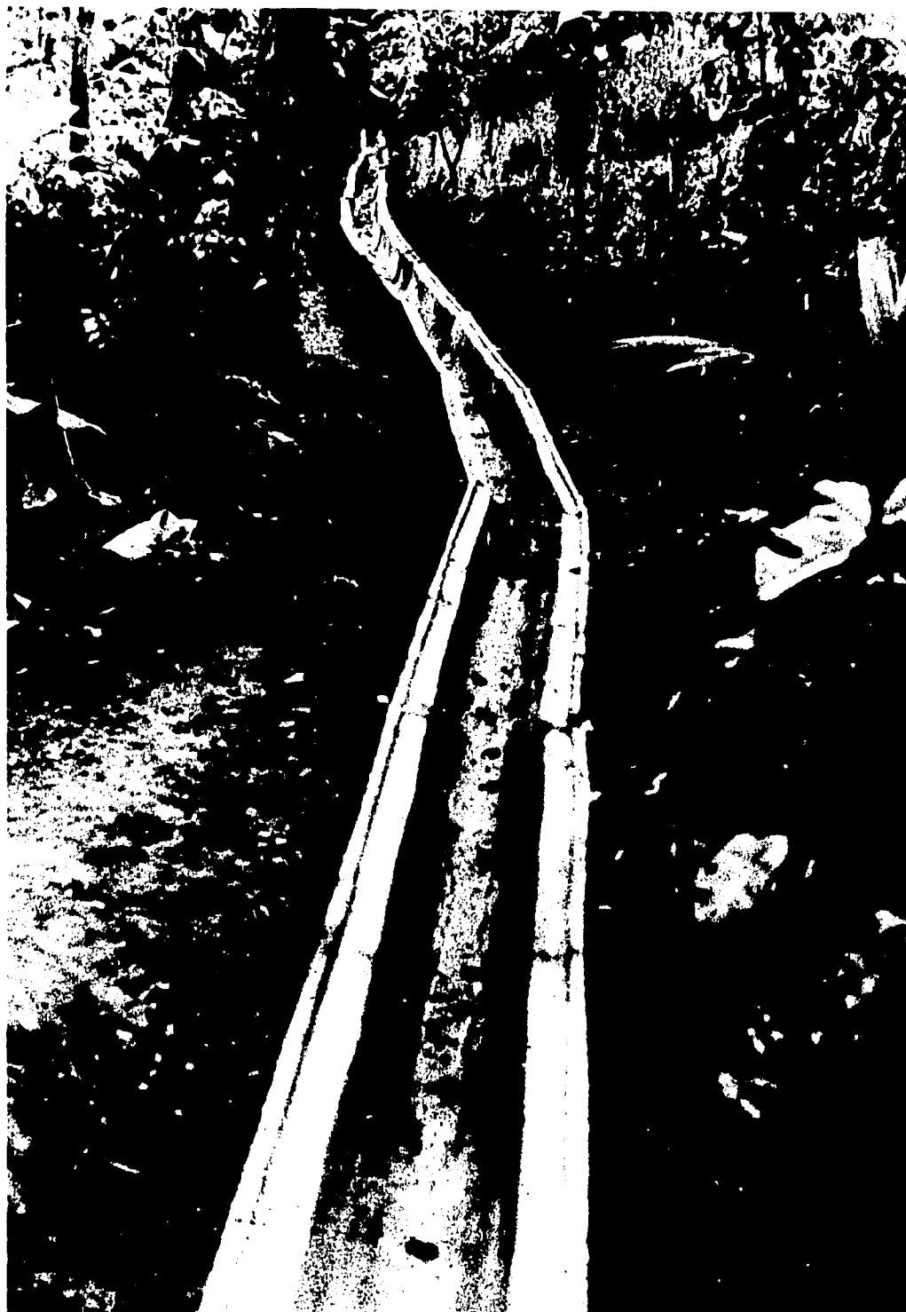
Figure 24 FERROCEMENT CHANEL IN LINE AS DISTRIBUTION SYSTEM
