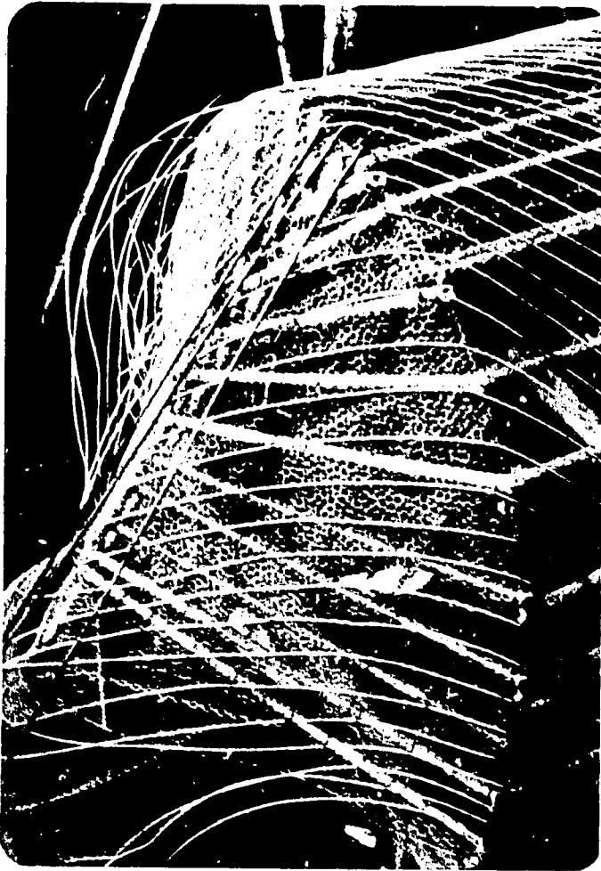
Figure 29 REINFORCEMENT OF PONTOON
