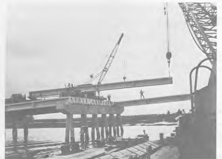
A major bridge under construction northeast of Saigon.
