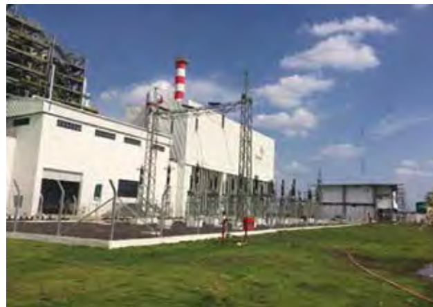
Figure 6.19: Waste-to-energy plant site in Jabalpur, Madhya Pradesh
