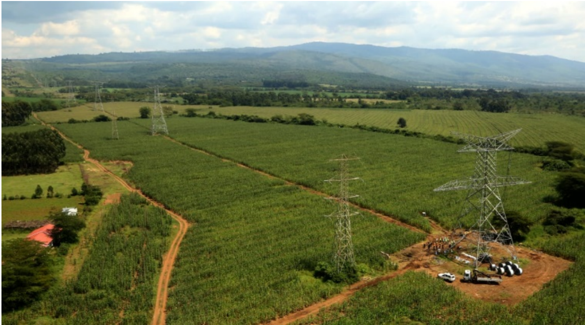
Olkaria–Lessos–Kisumu transmission line, Kenya. Photo credit: Nyaga Ileri
