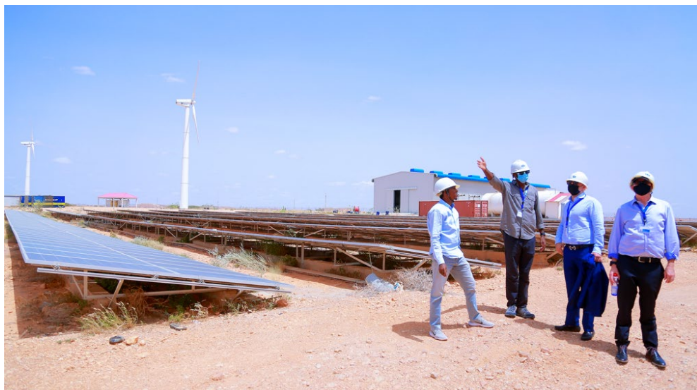
EAEP team visiting NECSOM power plant for diagnostics. Photo credit: EAEP
