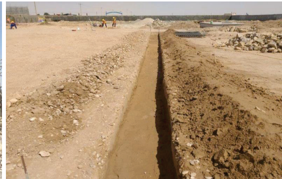
Photo #6: Excavation of roadside ditches, Mazar-e-Sharif, Balkh Province. ZA, 2021-05-22.
