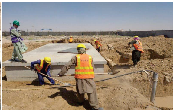
Photo #4: Backfilling of water reservoir, Mazar-e-Sharif, Balkh Province. ZA, 2021-05-20.
