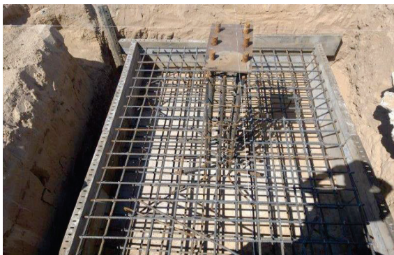
Photo #3: Installing foundation formwork, Mazar-e-Sharif, Balkh Province. ZA, 2021-05-19.
