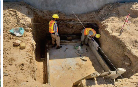
Photo #2: Installing foundation formwork, Mazar-e-Sharif, Balkh Province. JB, 2021-05-19.
