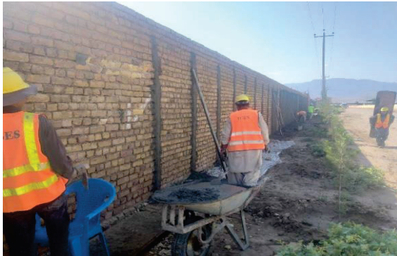
Photo #1: Plastering of perimeter wall, Mazar-e-Sharif, Balkh Province. ZA, 2021-05-18.
