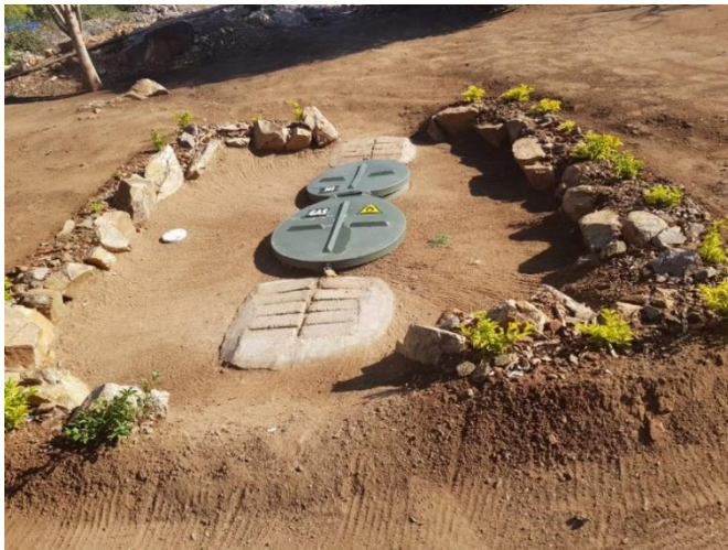
Photo 10: An inserted biogas system at Takheleni Primary School in Mpumalanga.
