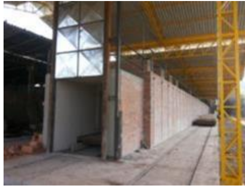
Figure 19 Completed Hoffman kiln at Sugres
