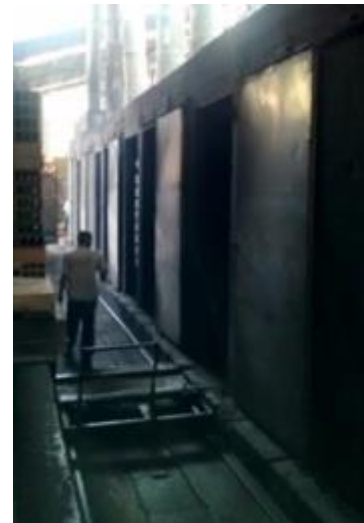
Figure 22 Improvements to doors in drying area at Delta
