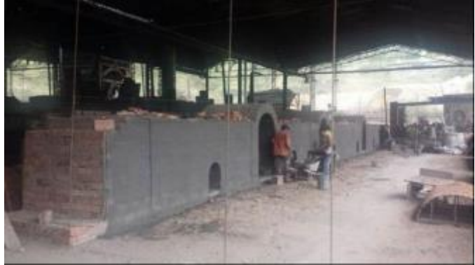
Figure 21 Construction progress at Pueblo Viejo (Partial view)
