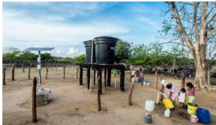
Figure 15 - Solar water pumping completed in Guajira
