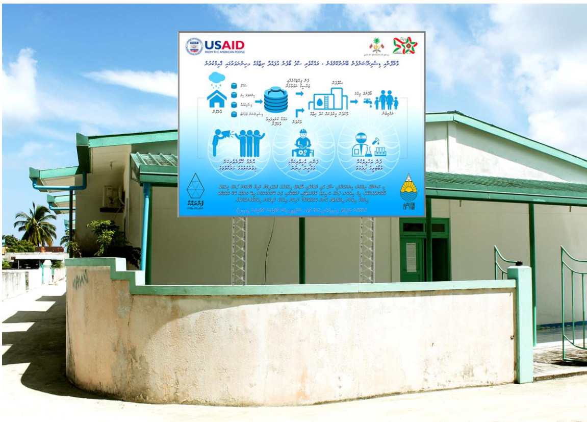
A GCC-produced billboard explains the integrated water system being constructed in Hinnavaru.
