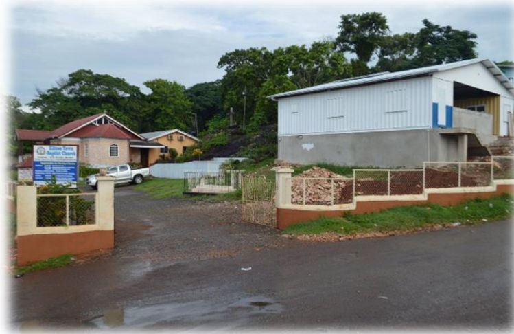
View from outside the Kitson Town CRC as it approaches completion.
