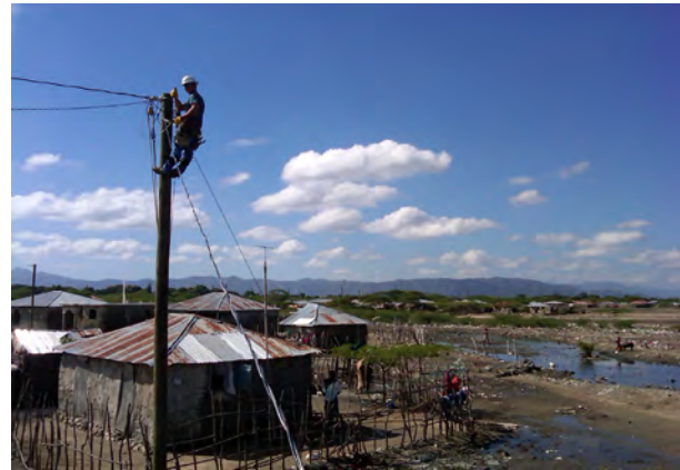
Figure 16: Connecting a customer in Caracol commune
