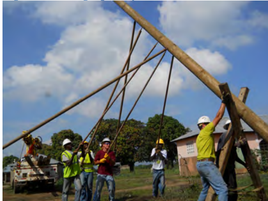
Figure 6: Setting a pole by hand
