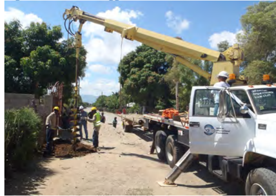
Figure 5: Donated digger derrick in Lombard
