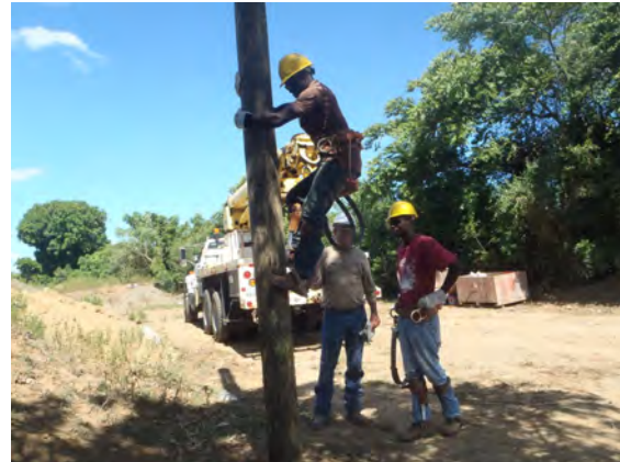
Figure 13: First time up a pole: CCEP lineman learns pole-climbing techniques
