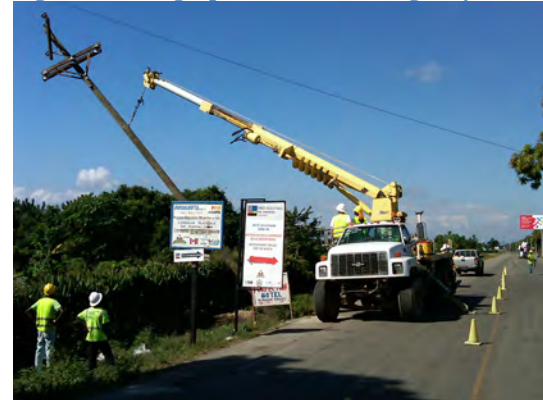
Figure 7: Setting a pole on National Highway 6
