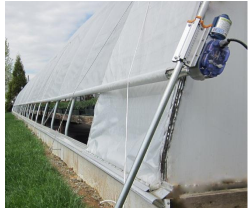
FIGURE 1 MOTORIZED ROLLUP SIDEWALL CURTAIN
