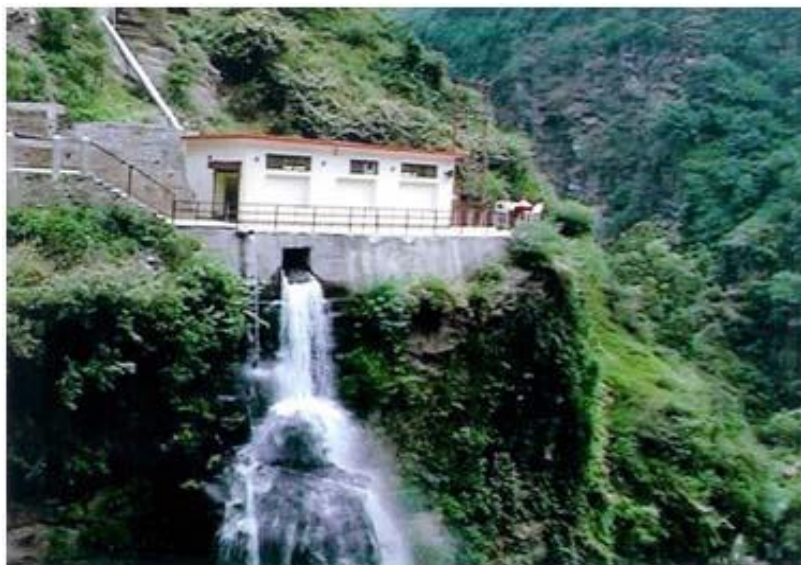
Ghandruk Micro-Hydro Power Plant
