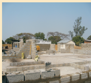
Building foundation for new pharmacy
