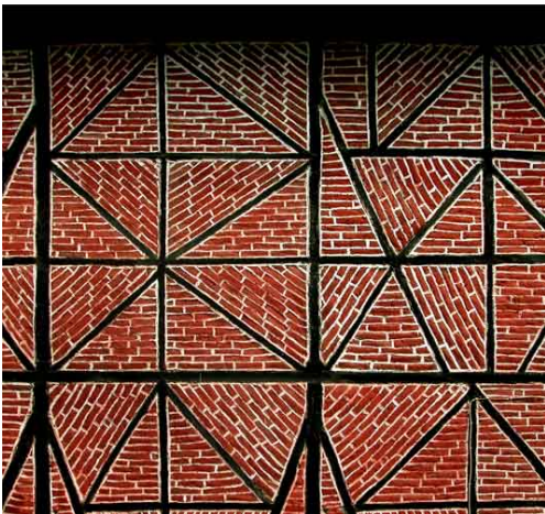
Figure 16. Detail of Ornate Variation of Hımiş Construction near Düzce (Gülkan and Langenbach, 2004)
