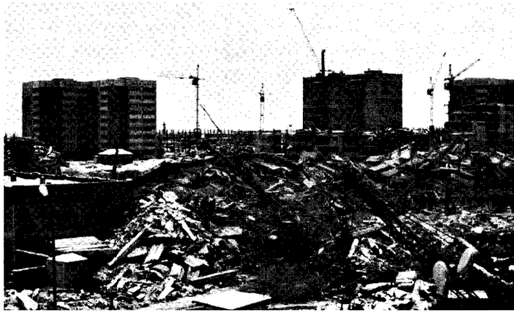
Figure 7. Precast Frame Type Building Collapses in the Foreground and Large Panel Buildings in the Background, 1988 Spitak (Armenia) Earthquake (Earthquake Spectra (1989), Special Issue on the Armenian Earthquake, 5_S1 (August))
