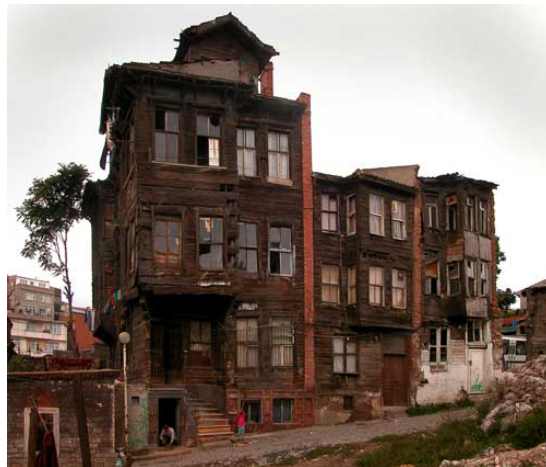
Figure 17. Nearly Derelict Row of Timber Houses in the Fatih District of Istanbul (Gülkan and Langenbach, 2004)
