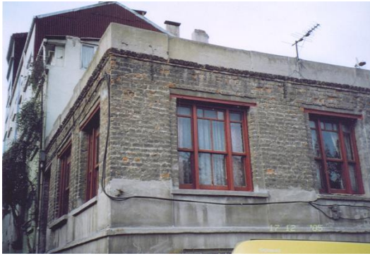
(a) Unreinforced Solid Brick Masonry
