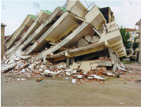
Figure 8. Reinforced Concrete Frame Collapse (Turkey)
