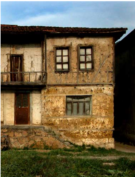
Figure 15. Dwelling with Hatils in the Masonry Bearing Ground Floor Walls, and Himiş Construction Above, Turkey (Gülkan and Langenbach, 2004)
