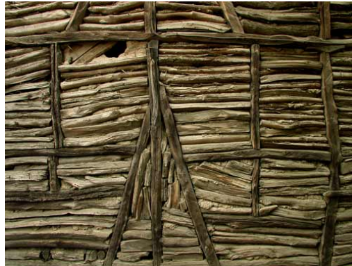
Figure 18. Detail of Bağdadi Wall, Gölcük
