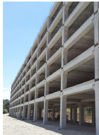
Figure 5. Components of a Precast Reinforced Concrete Frame Building ( http://theconstructor.org/concrete/structural-uses-of-precast-concrete/6289/ )
