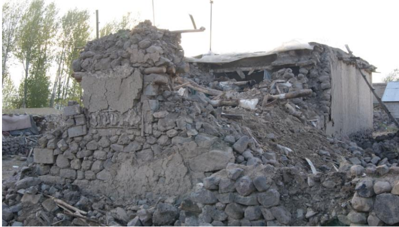
Figure 1. Vernacular Rural Stone Masonry Architecture, Van Earthquake, 2011 ( http://eerc.metu.edu.tr/tr/system/files/images/vaneq2310/van_odtu_dmam_rapor.pdf )
