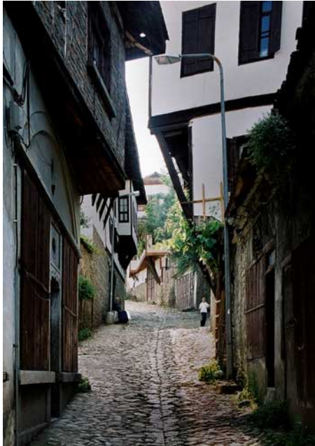
Figure 14. Street of Houses with Overhanging Jetties of Himiş Construction (Gülkan and Langenbach, 2004)
