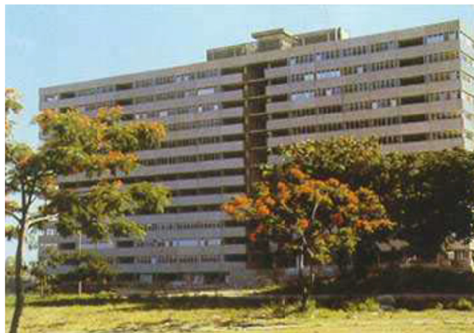
Figure 4: A typical precast slab-column building (WHE Report #68, Serbia and Montenegro)
