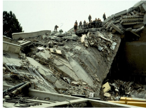
Figure 9. Reinforced Concrete Frame Collapse (Mexico)
