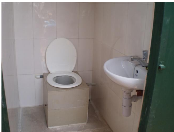
Picture 3: Wastewater from Hand-washing Used for Flushing
