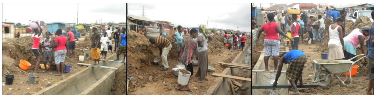
Picture 5: Community participation in backfilling of drain construction in Avenor
