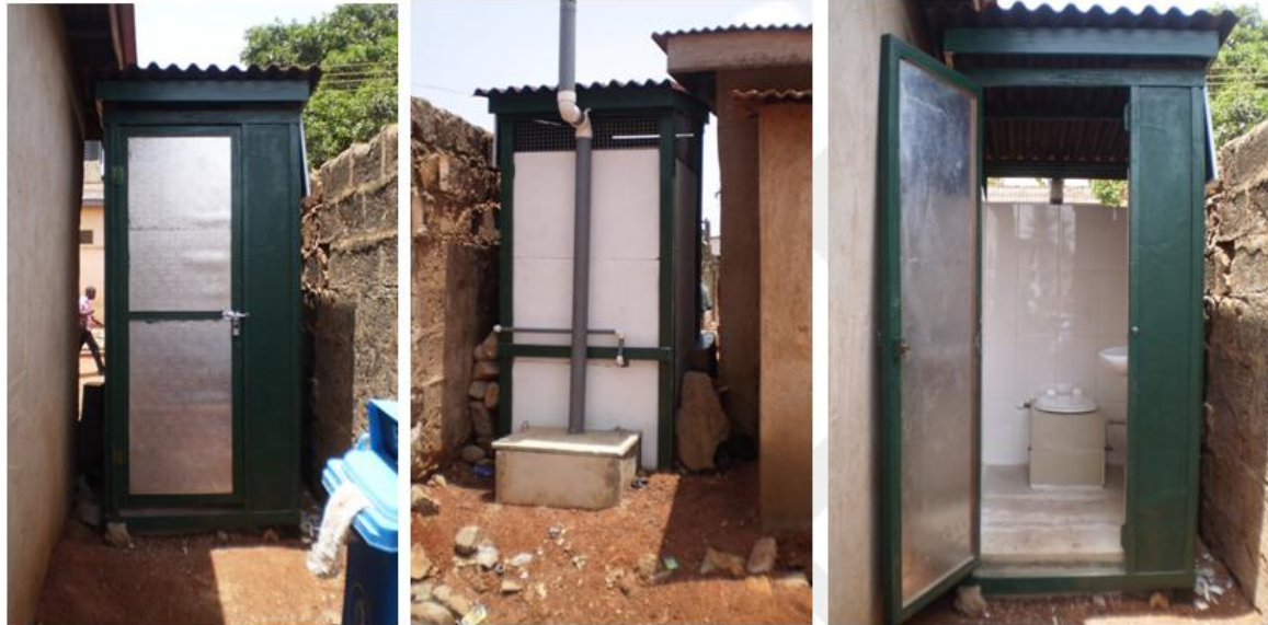
Picture 2: Front & Back views of A Biofil Latrine Showing Digester
