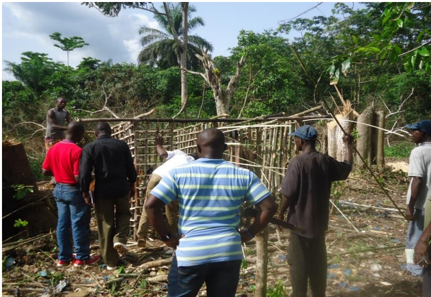
Global Communities staff monitoring CLTS structures in Panta-Kpaai District
