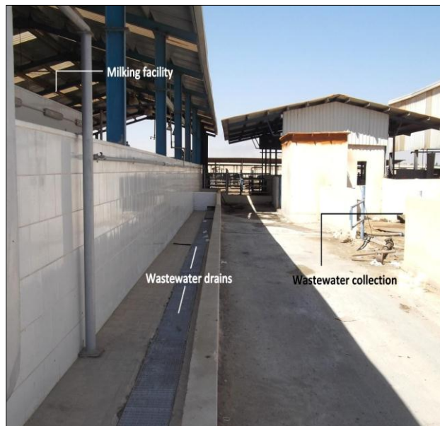
Figure 3-1: A milking facility, drains to wastewater collection/prereatment/disposal
