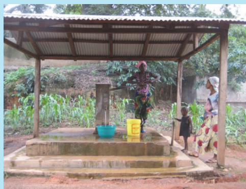
Clients at the Regional Hospital of Faranah use the water pump, which was built after the SBM-R process pointed to the need for an on-site water source.
