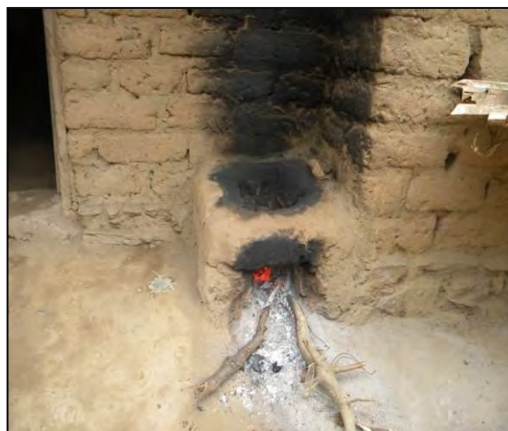
A fuel efficient built-in stove promoted by the project.
