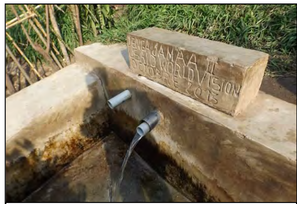
Example of a capped spring
