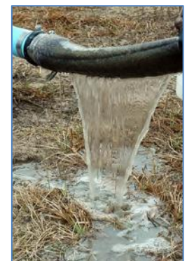
Figure 9: Cloth filter bag attached to inlet pipe
