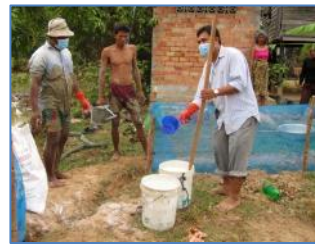
Figure 5: Mixing burnt lime in a bucket
