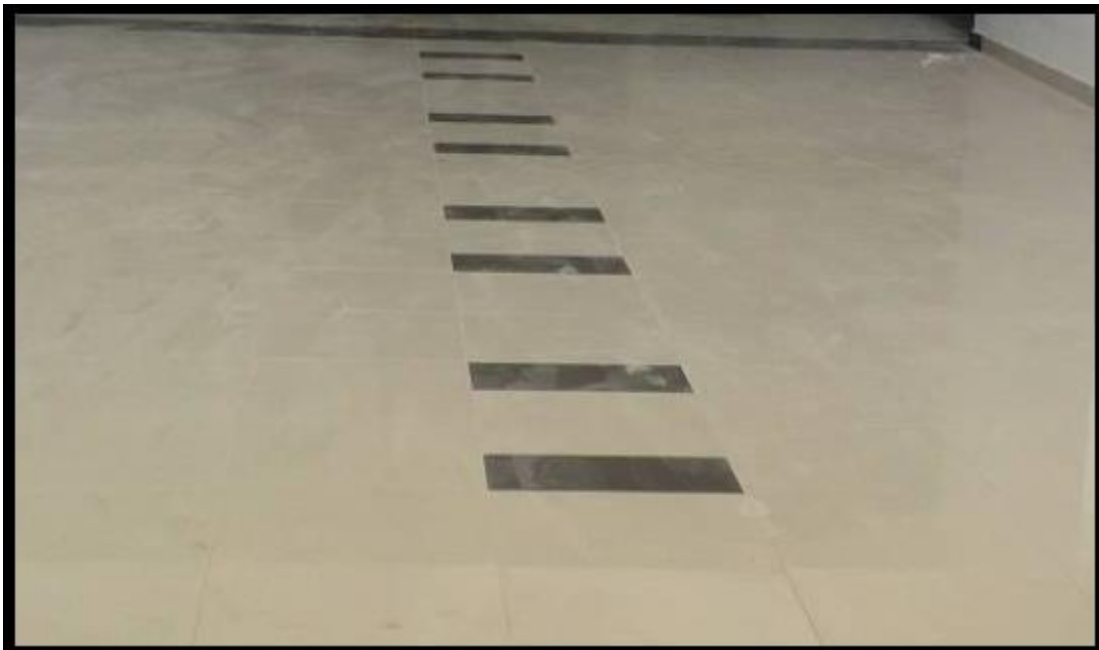
Figure 11 Tiles Installed for Flooring at the Under Construction Buliding in Islamabad
