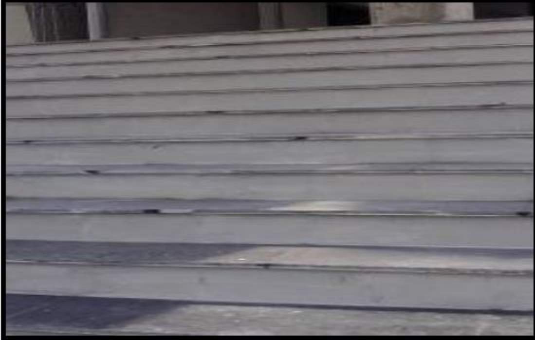
Figure 10 Granite Being Installed At the Steps of an Under Construction Buliding in Islamabad
