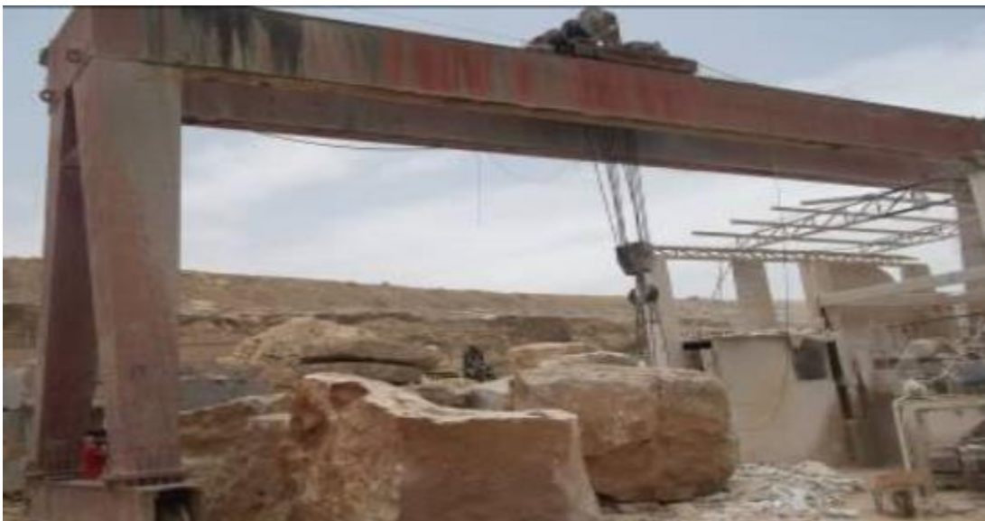
Figure 20 A Crane Being Used to Lift Loads beyond Its Rated Capacity
