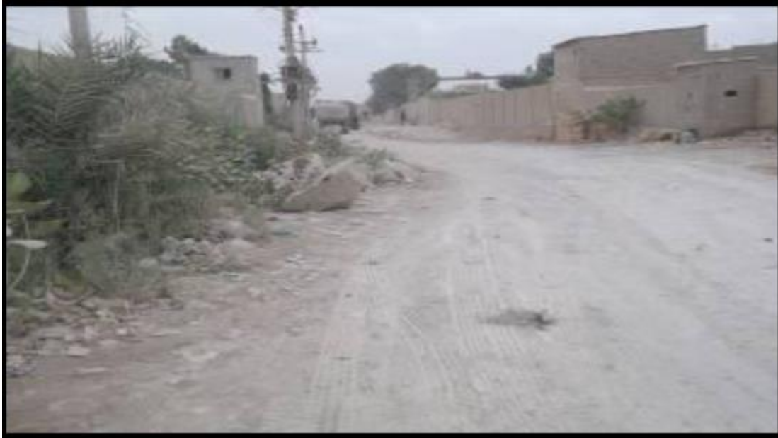
Figure 27 Poor Conditions of the Road near Manghopir Road, Where Most of the Processing Units Are Located
