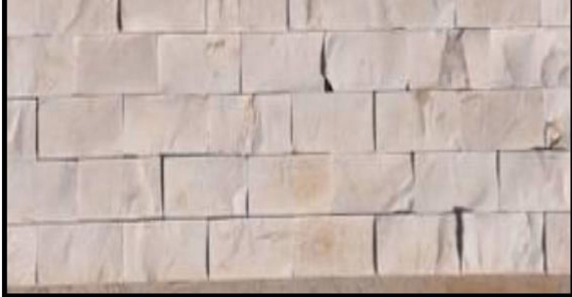
Figure 15 Split Face Finishing for Wall Cladding
