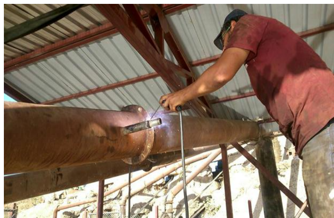
Worker installs pipes inside the new pumping station.
