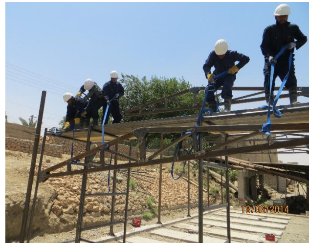
Syrian subcontractors raise the steel beams of the pumping station.
