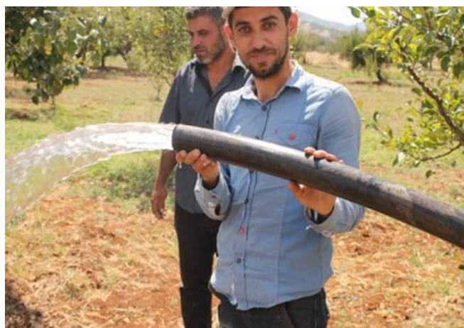
Water flows from solar powered irrigation pumps installed by the ES-North project in Syrian apple orchards.
