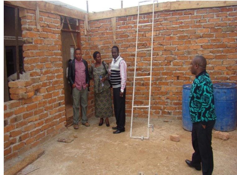
View of the construction of patient waiting bay in Kilolo H/C
