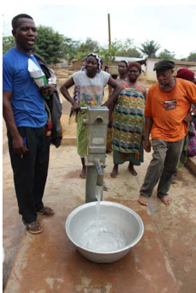
Demonstrating the strength of a repaired borehole facility.
