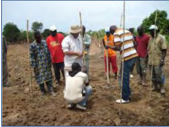
Volunteer Joe Sullivan demonstrating pond construction techniques
