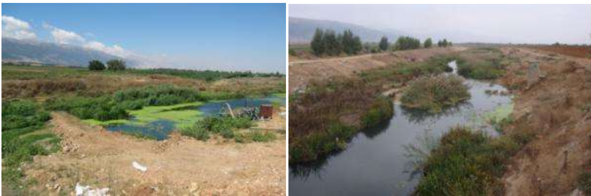
Riverbed dammed for irrigation pumping (Ghazze), Over-widened riverbed but not maintained (Joub Jenine) regardless of water quality
