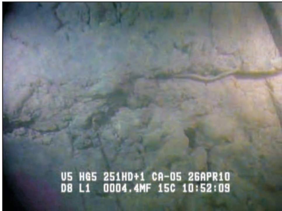
Image 1-18: 2010-04-26-1052 - Porous concrete interface on spillway.
