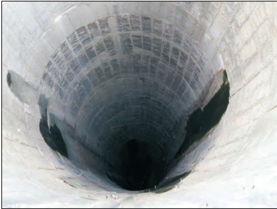
Image 4-9: View down small spillway riser.
