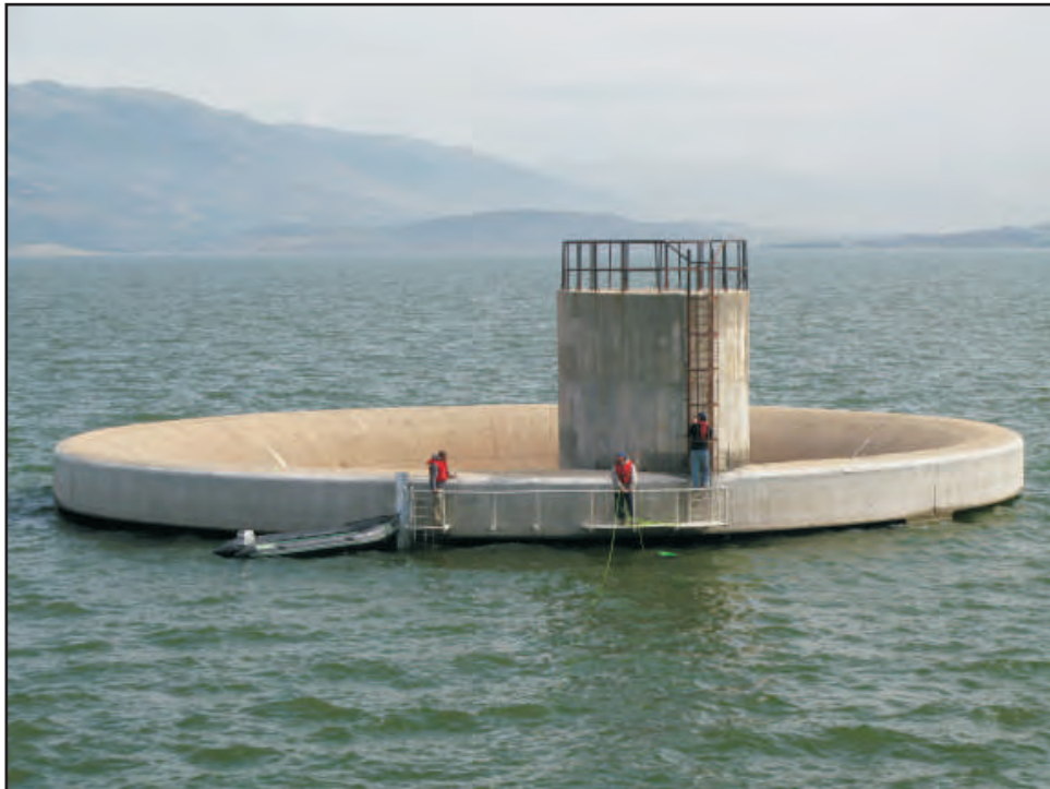
Image 4-8: Accessing the spillway structure.
