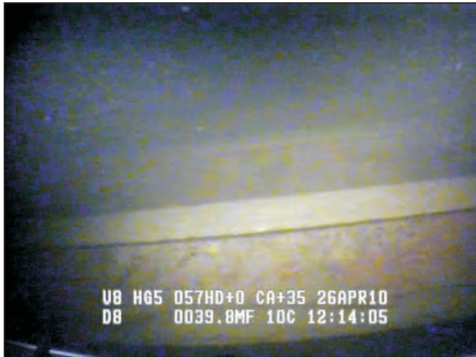
Image 1-21: 2010-04-26-1214 - I-Beams leading south from intake.
