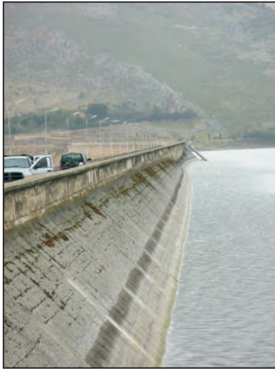
Image 4-5: View looking west along dam face showing bend to south.
