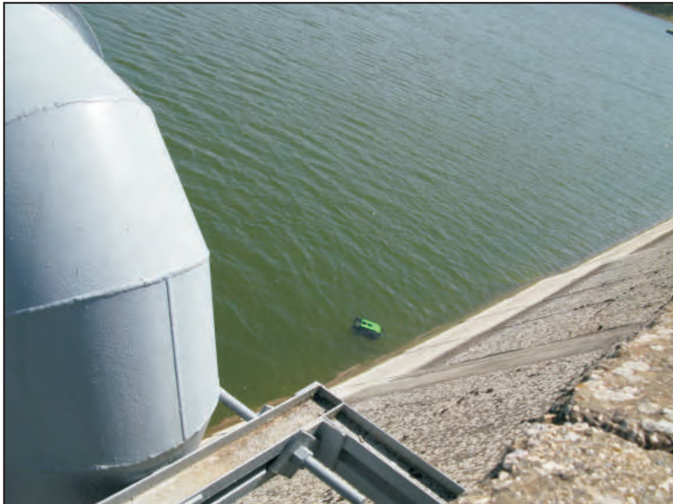
Image 4-2: ROV near vent pipe.
