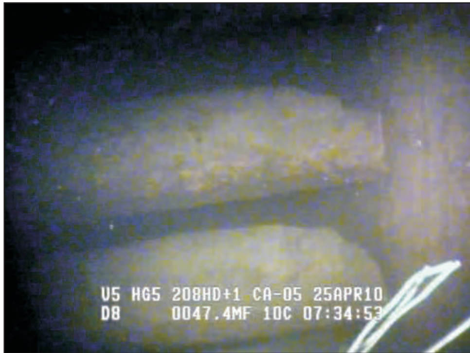
Image 1-13: 2010-04-25-0734 - Horizontal vanes in power tunnel inlet.
