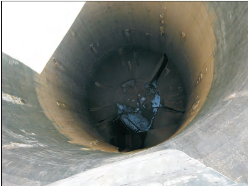
Image 4-10: View looking down large spillway riser.
