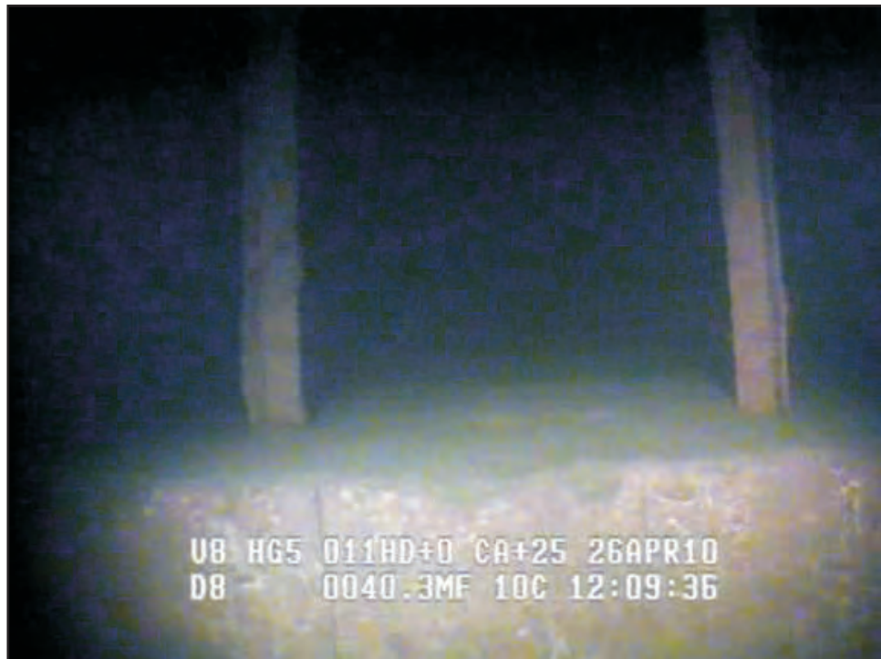
Image 1-20: 2010-04-26-1209 - Top of irrigation intake.
