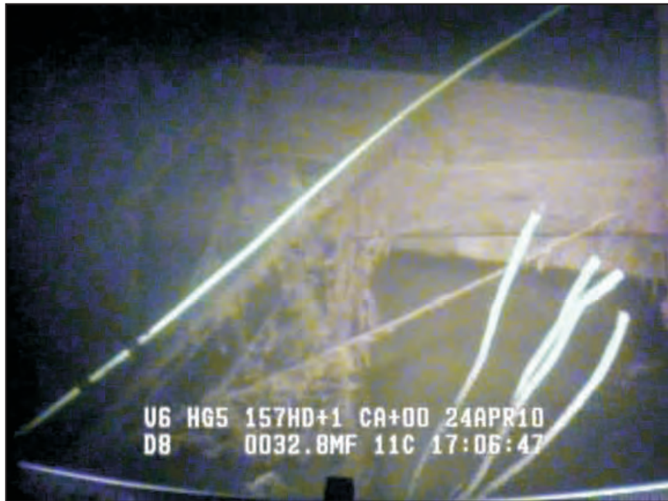
Image 1-9: 2010-04-24-1706 - Net, ropes and debris hanging on platform near joint 10 at elevation 815 m.
