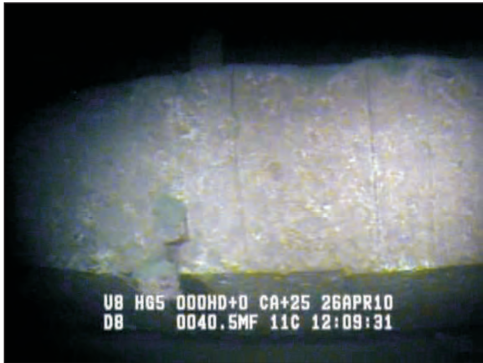
Image 1-19: 2010-04-26-1209 - Irrigation intake structure.
