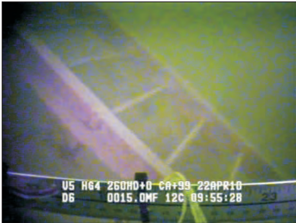
Image 1-5: 2010-04-22-0955 - Ladder at vertical joint 21.
