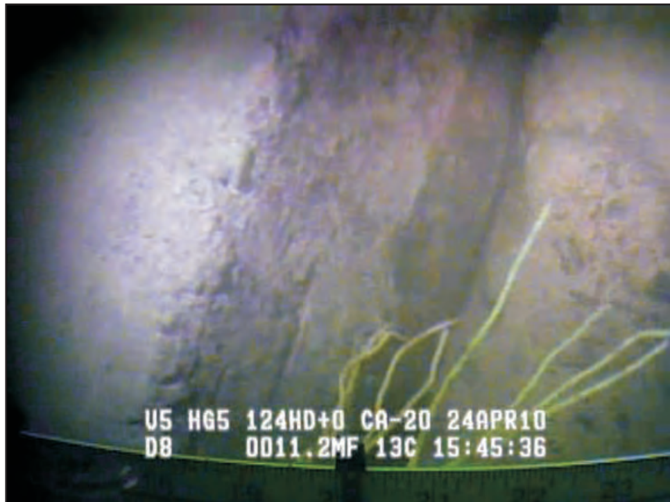
Image 1-8: 2010-04-24-1545 - Raised slab at joint O2.
