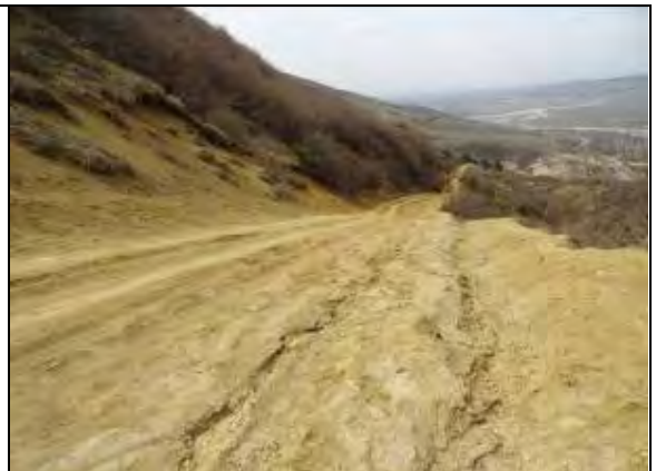
Erosion is a typical pattern all along the route.
