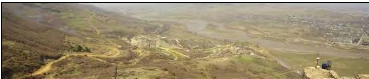
Scars in the landscape are essentially the Gorijvari road. Erosion is significant across the entire section and locals inform (and is evident from site inspection), that downhill movement of the water during storm events should be a significant factor in completing the road design.
