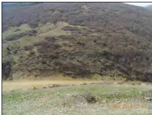
Site #132 Landslide at the upper end of road
