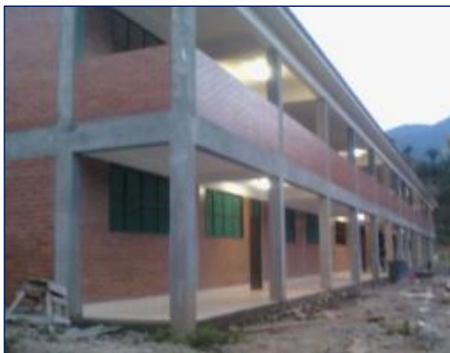
The Rene Barrientos Ortuño School building almost finished, in La Asunta.
