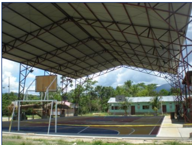
The multi functional sports complex with roof in Santa Ana de Mostenes.
