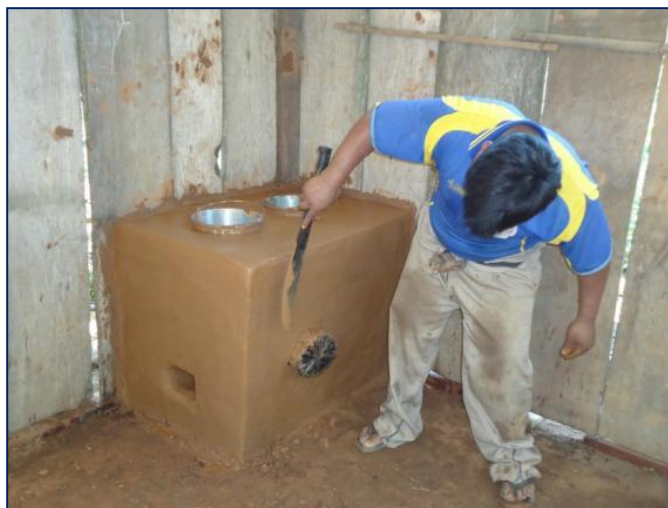
A community member constructing a stove.
