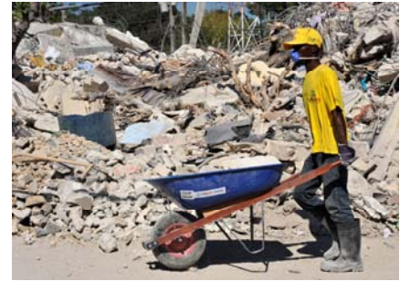
A CFW beneficiary conducts rubble removal activities. (Photo: USAID)
